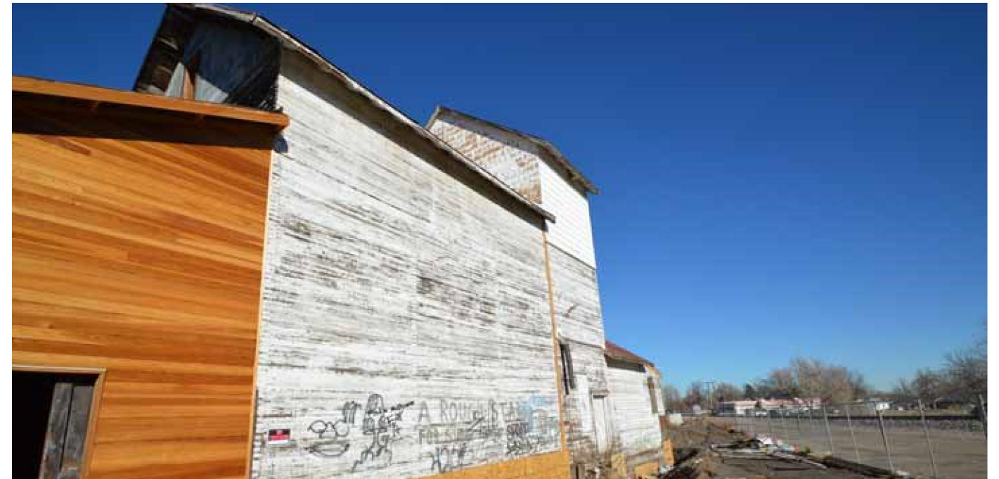
Louisville Grain Elevator
