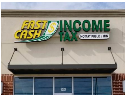
Exposed raceway
