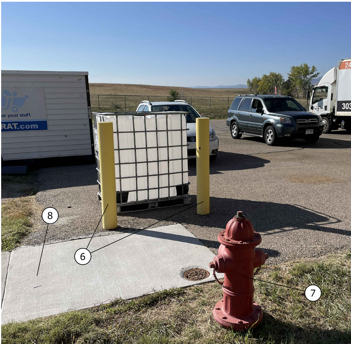
EXISTING FIRE HYDRANT AND BOLLARDS
