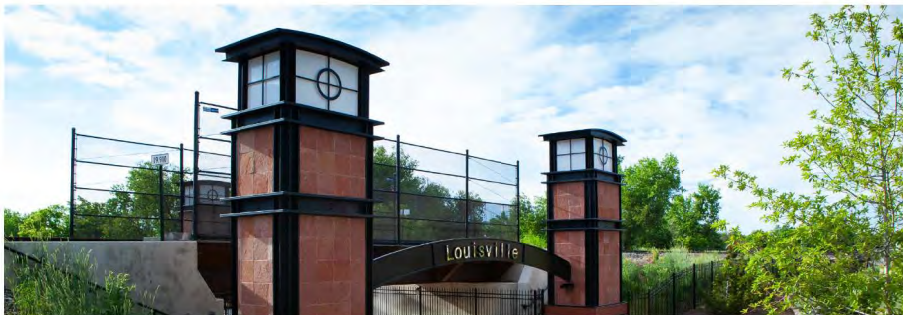
South Street Underpass Source: City of Louisville
