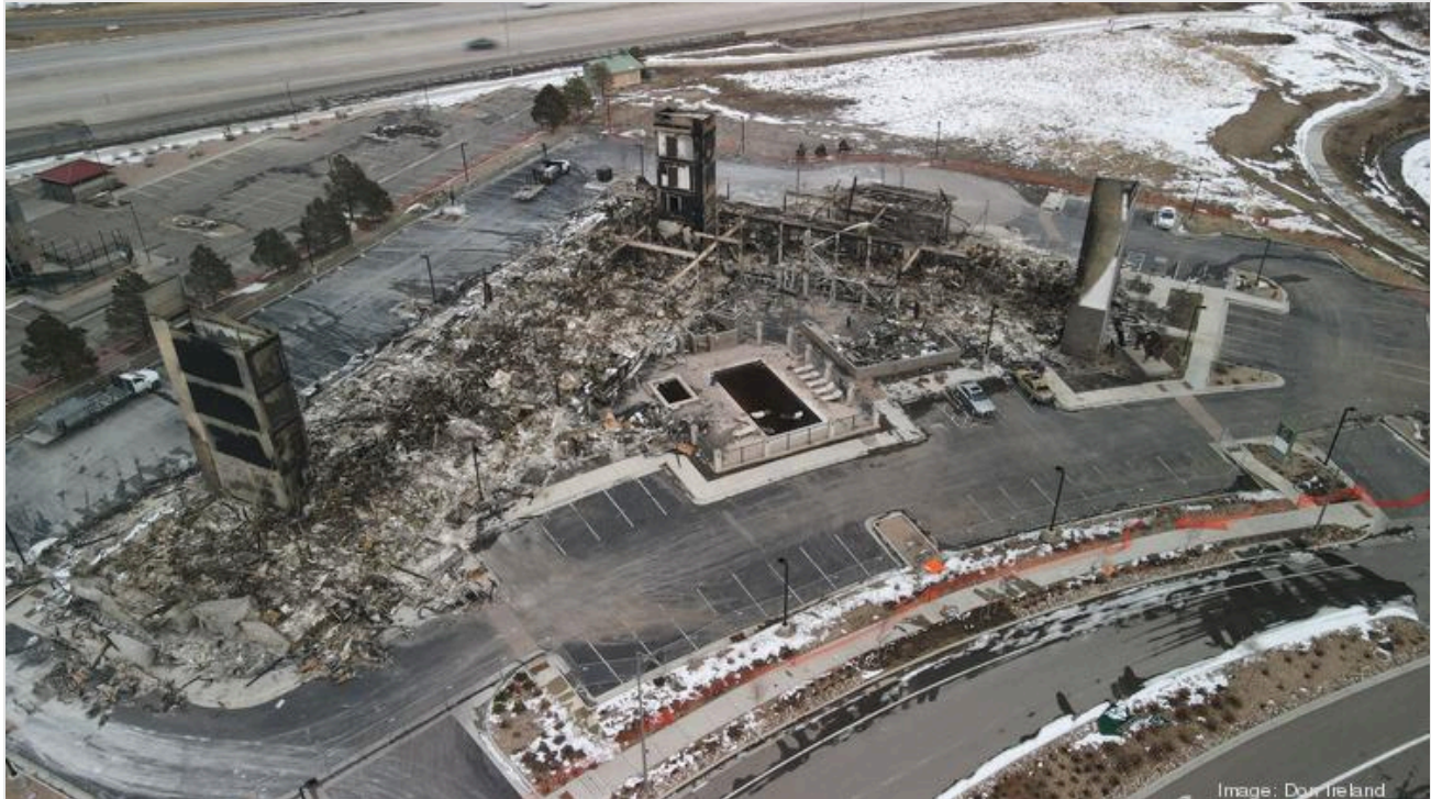
Remains of Element Hotel in Superior following the Marshall Fire.
