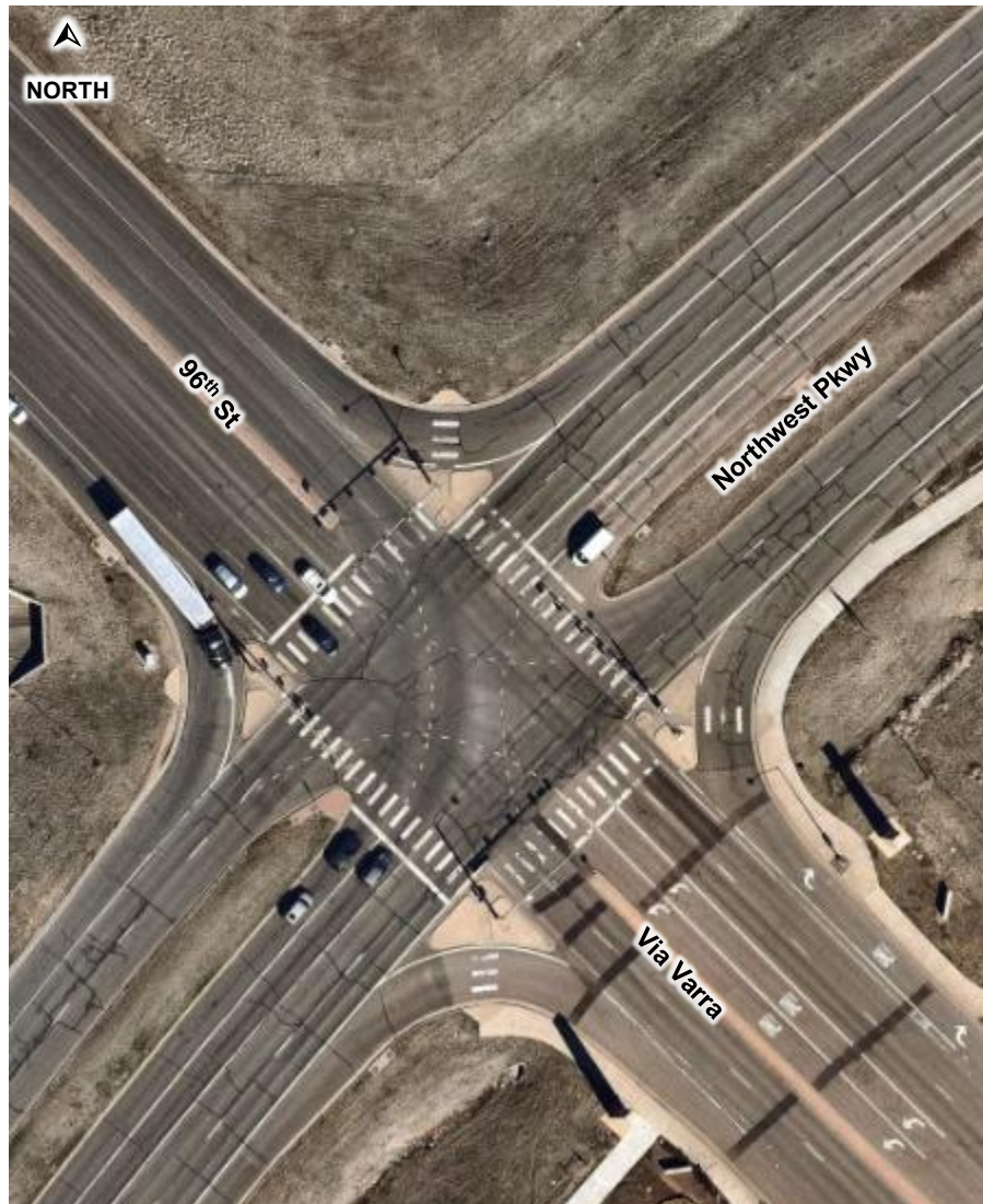
96 th Street/Via Varra & Northwest Parkway (#2)
