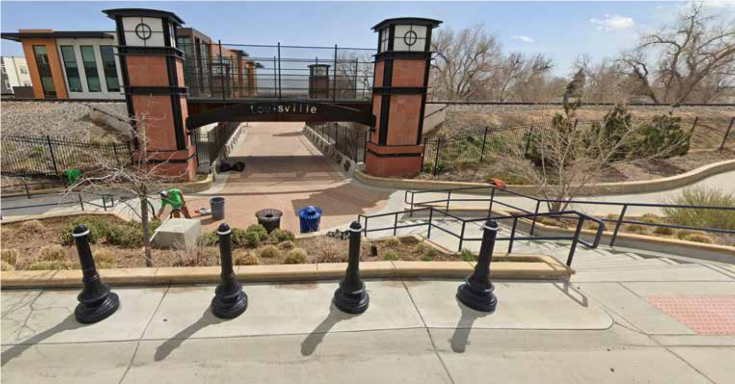
Figure 1. South Street Underpass (Source: Google Maps)
