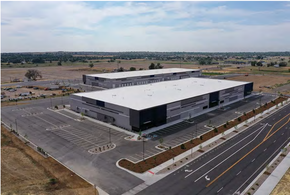
Solid Power headquarters.
