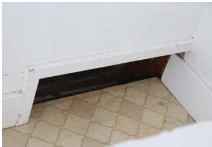
Image 3: Basement window is bisected by the main level landing to the basement stairs
