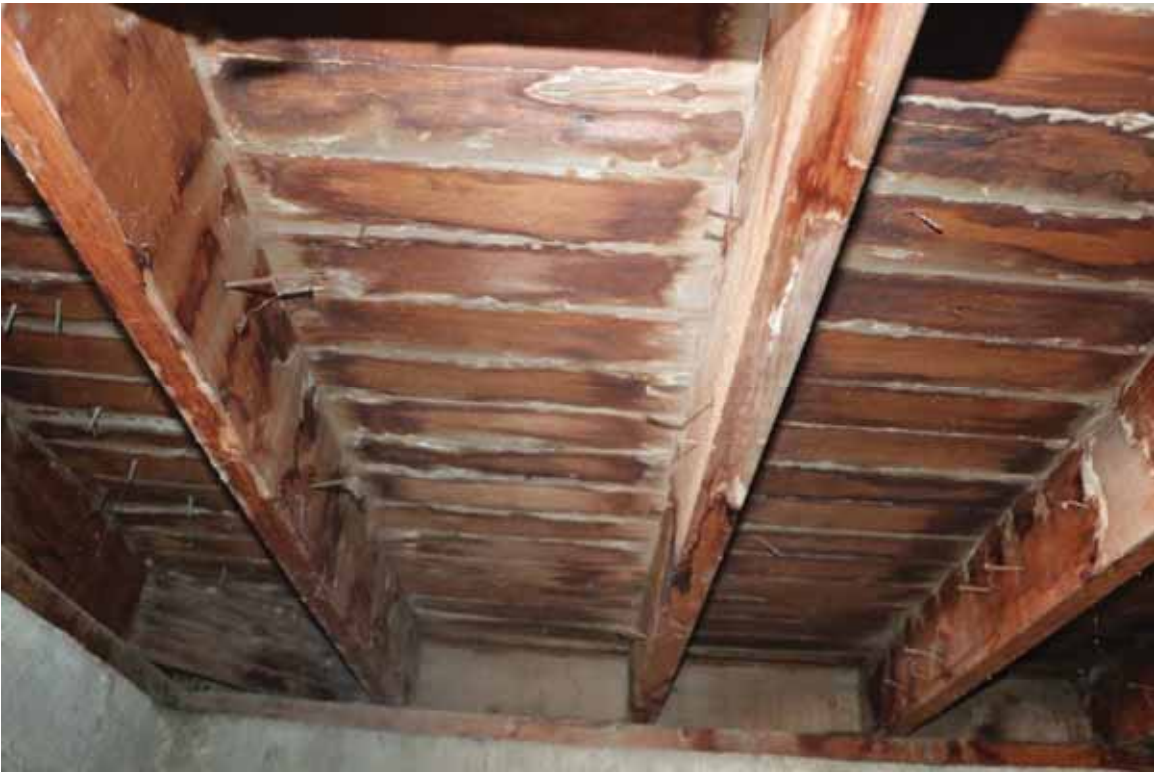
Image 18: Entry Porch_ Underside of porch floor
