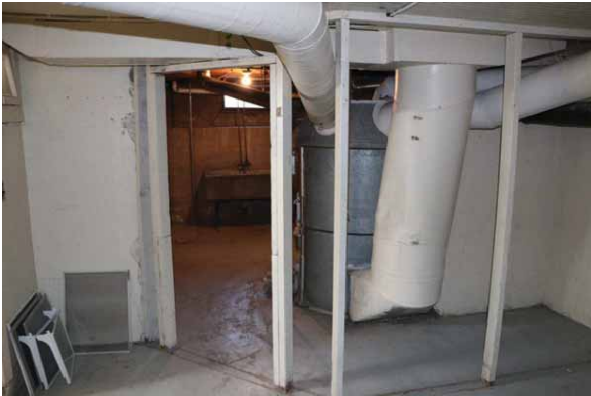
Image 37: Heating & Air-Conditioning_ Furnace ducting, return air at the bottom and distribution ducting at the top
