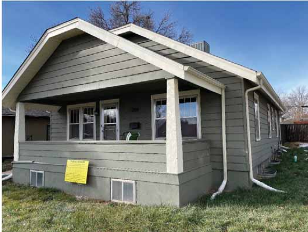
Figure 1: 1209 Main viewed from the northeast
