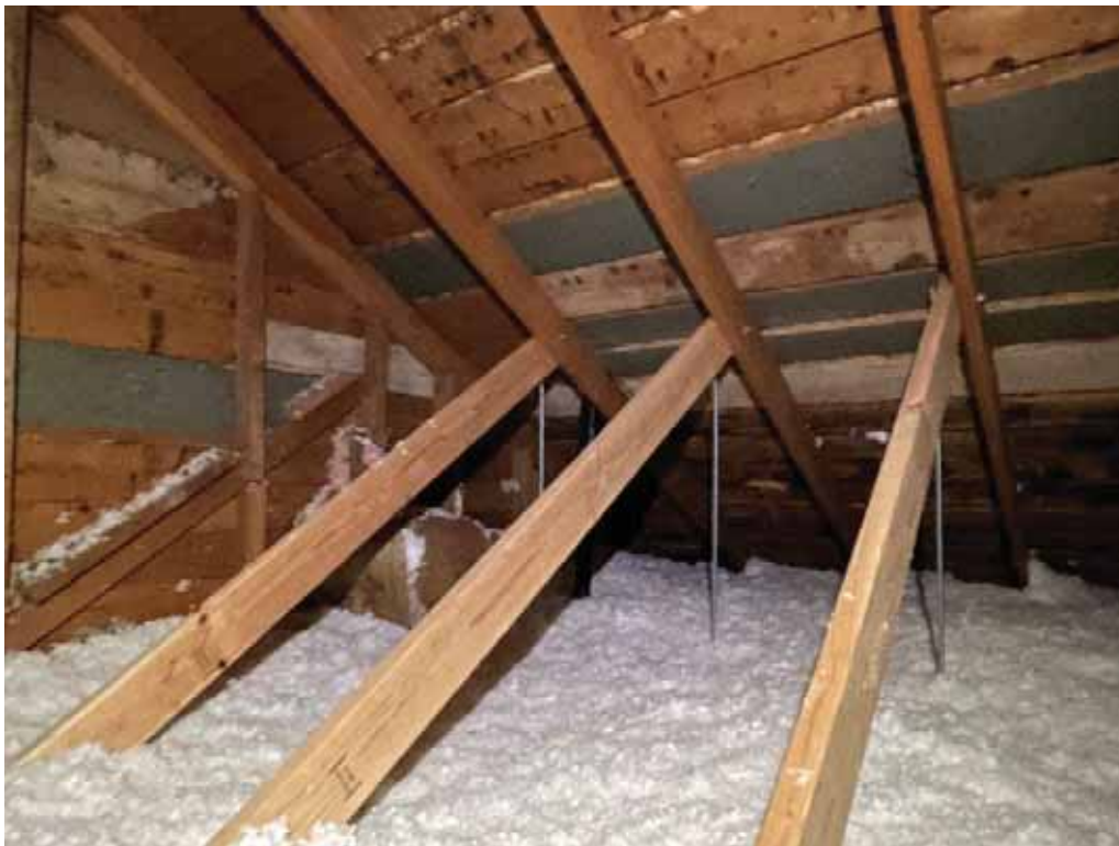
Figure 18: Discontinuous studs in west gable end wall
