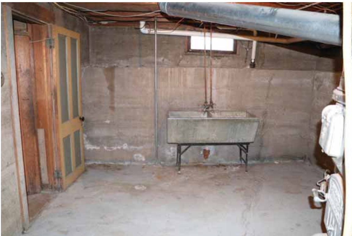
Image 11: Foundation Systems_ Poured concrete on grade with concrete walls. Stepped poured concrete foundation walls common throughout the basement
