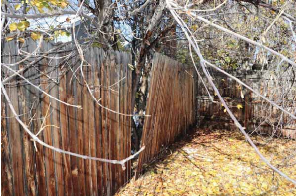
Image 10: Fencing Panel dislodged at west end
