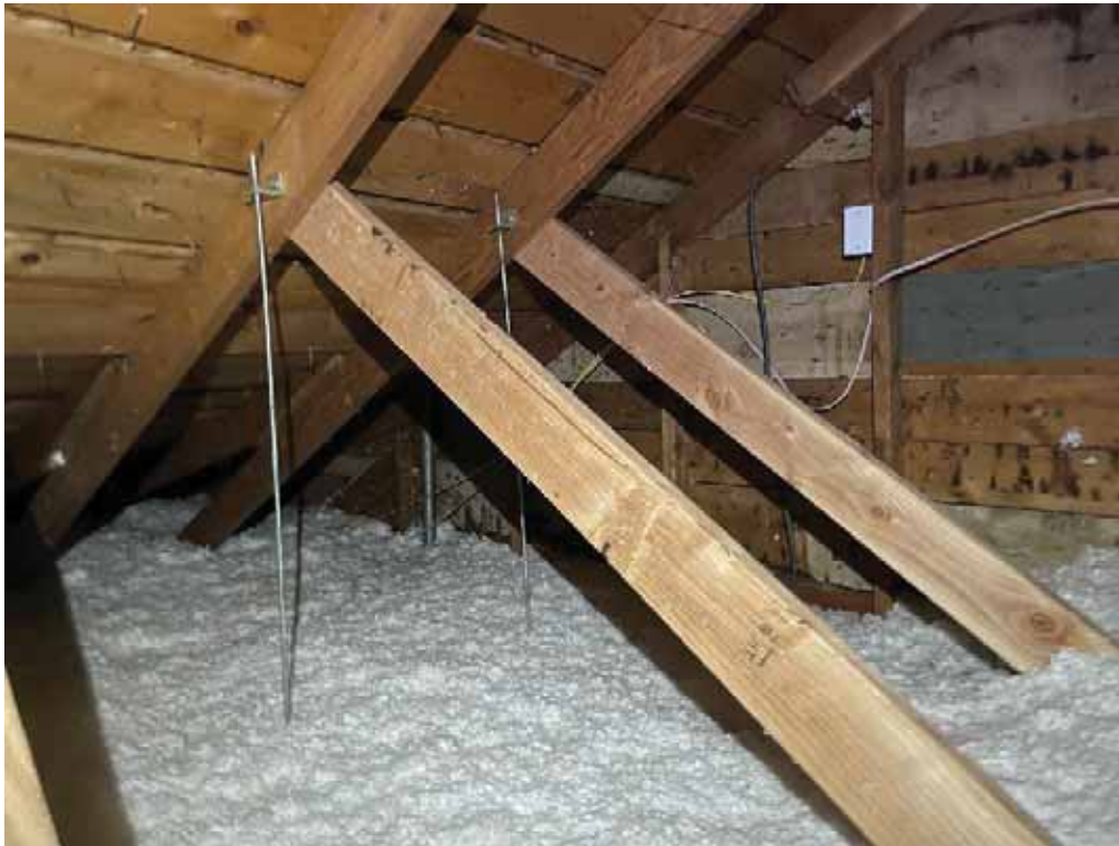
Figure 13: Roof framing with diagonal bracing and tie rod retrofit
