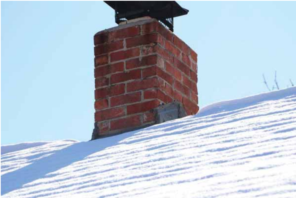
Image 21: Exterior Masonry_ Brick Chimney
