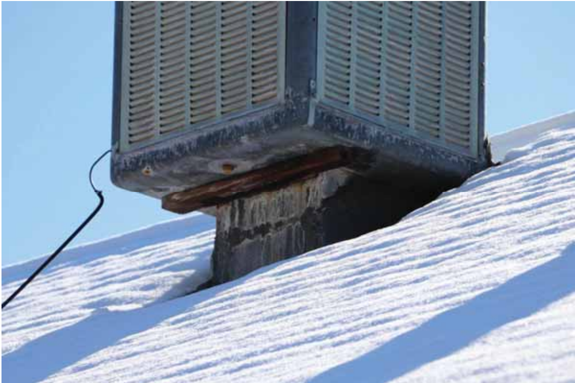
Image 22: Sheet Metal Flashing_ Swamp cooler flashing
