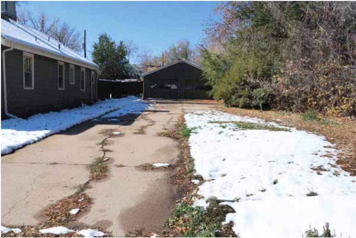
Image 9: Parking Concrete driveway
