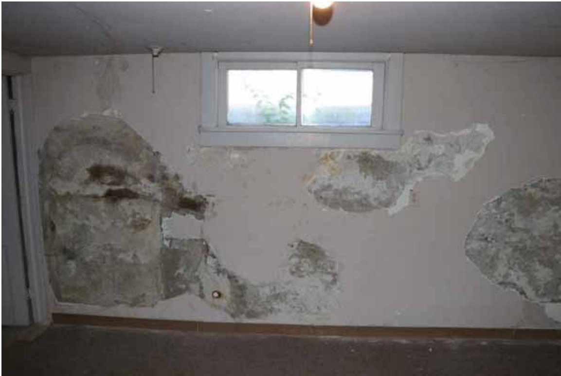
Image 12: Foundation Systems_ Sprinkler control box and hose bib are immediately adjacent on the exterior
