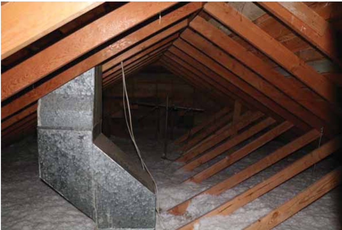
Image 14: Roof Framing Systems_ 2x6, 24"OC. View facing towards Main Street. Note the lack of purlins on the NE quarter
