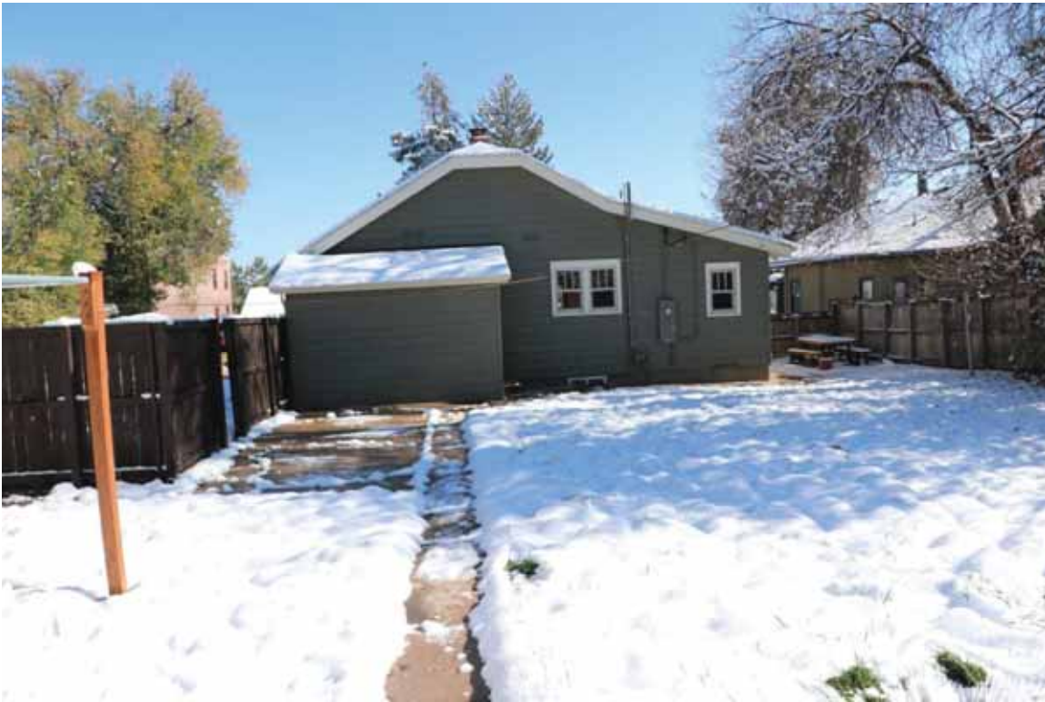
Image 7: Grading_ Lot slopes from rear of the home to the street. View facing towards Main Street
