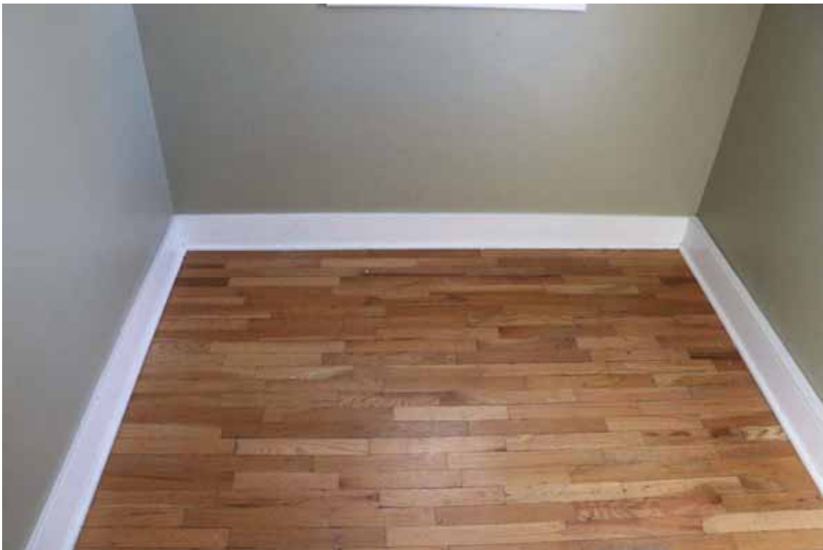
Image 33: Floor Finish Materials_ Representative wood floor and moulding
