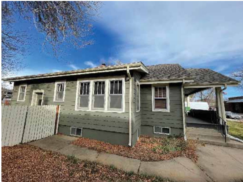
Figure 2: 1209 Main viewed from the south
