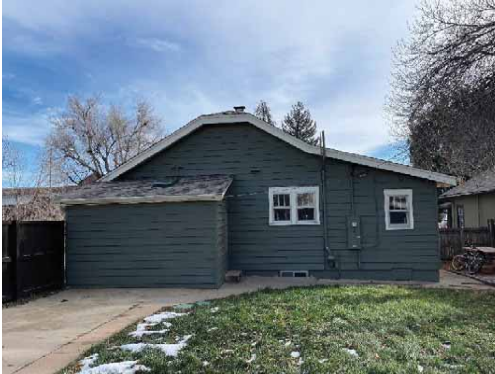
Figure 3: 1209 Main viewed from the west
