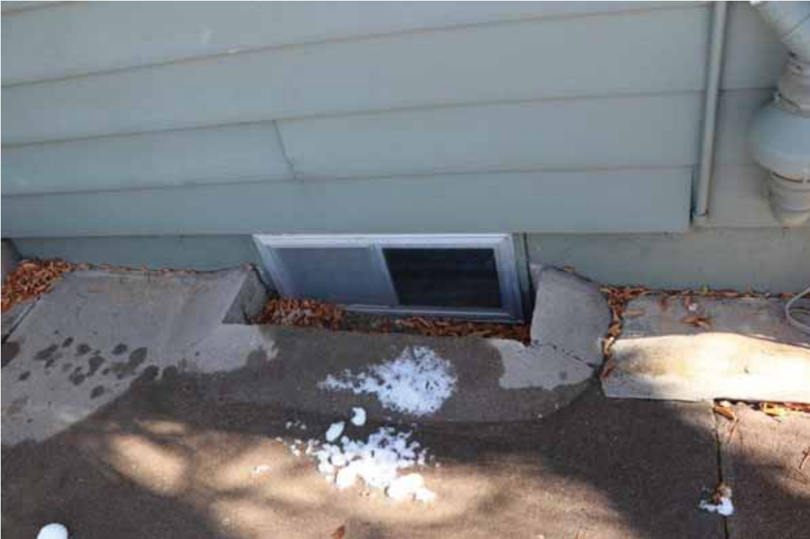
Image 8: Grading_ Lot slopes from rear of the home to the street. Curb around basement window
