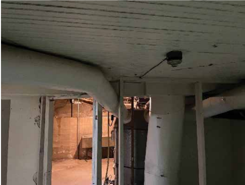
Figure 15: Stud wall at basement Room-2 supporting 2x8 floor joists with opening in concrete wall beyond
