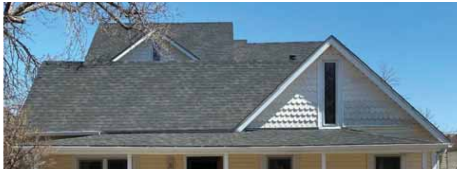
Asphalt composite shingle roof added in 2018
