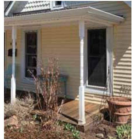
Covered front porch
