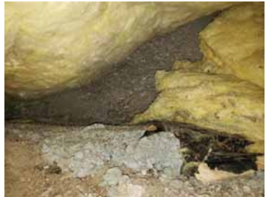
Crawlspace foundation with insulation pulled back
