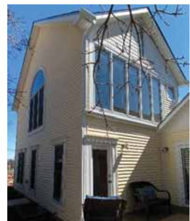
North & west side windows
