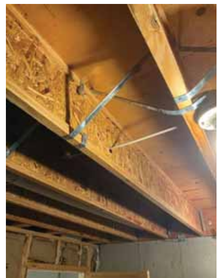
Floor framing in 1995 addition
