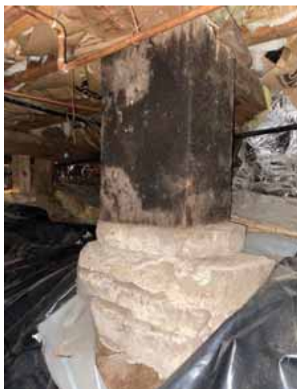
Support column in crawlspace
