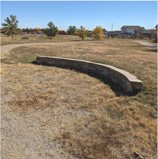
Existing Stone Wall
