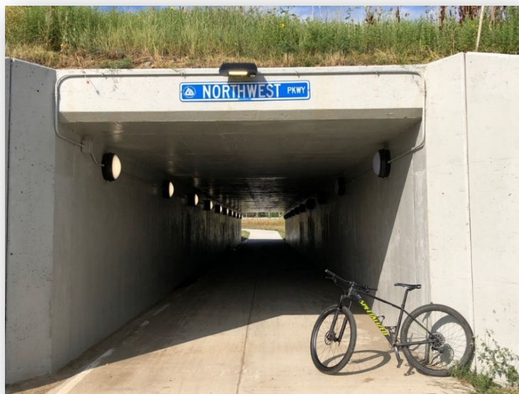
Figure 8. Northwest Parkway Multi-Use Path Underpass
