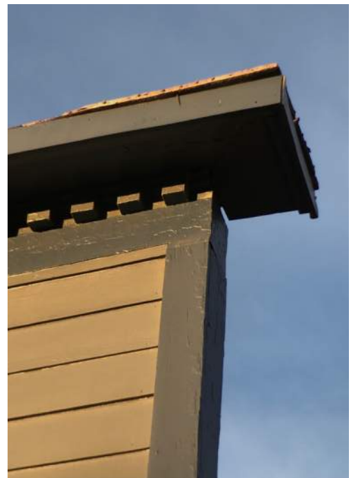
North façade cornice detail
