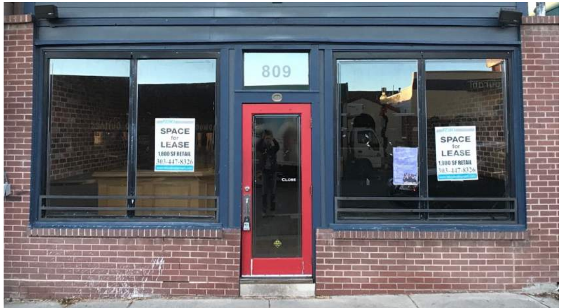
Exterior window and door detail
