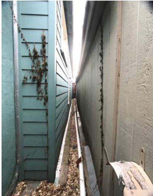
Detail of north exterior wall
