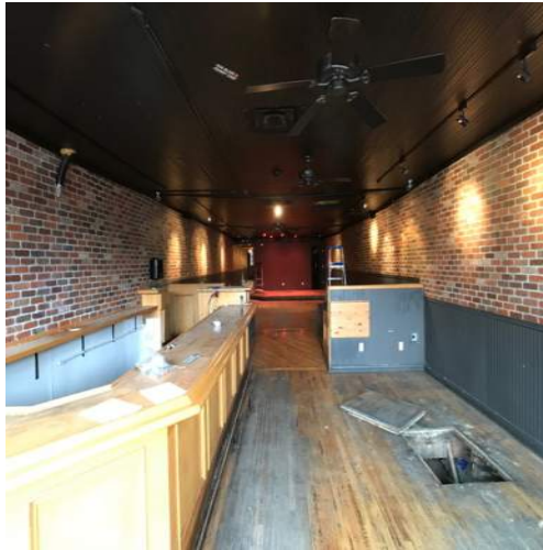
Interior detail of original building
