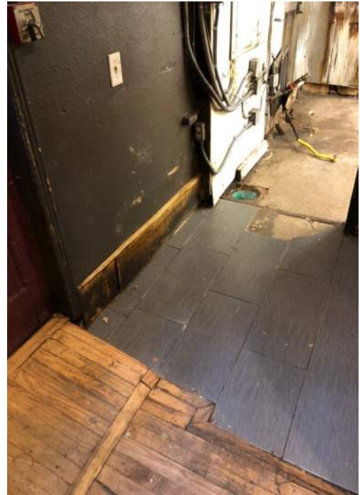
Concrete slab at kitchen addition
