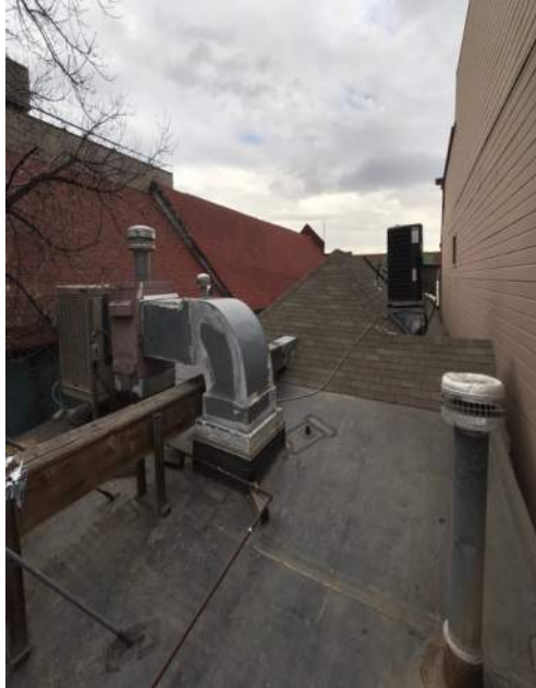
Membrane roof with penetrations
