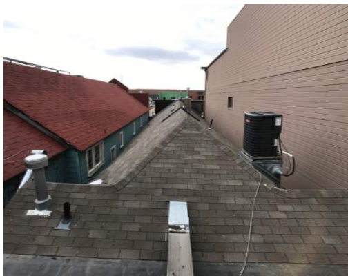
Asphalt shingles
