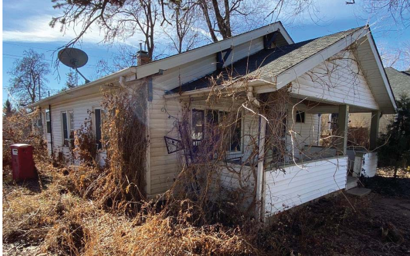
Northeast Corner looking Southwest
