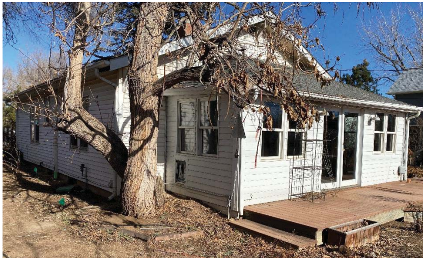
Southwest Corner looking Northeast
