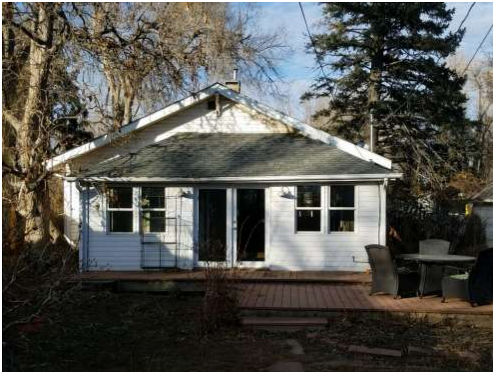
908 Rex Street, south view – Current Photo
